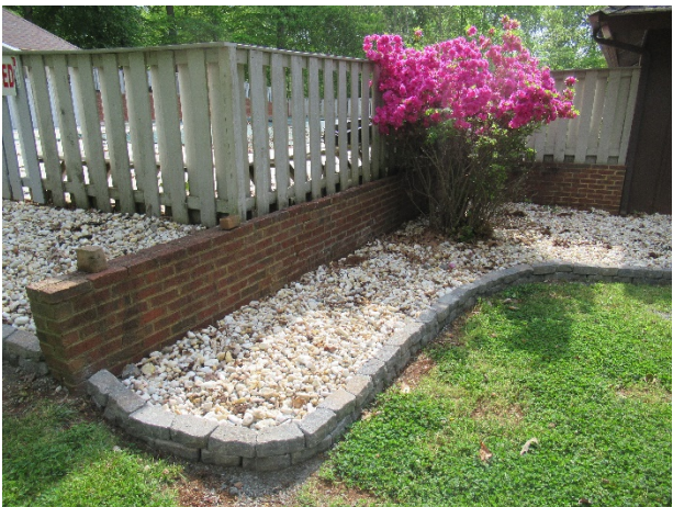
Masonry retaining wall overview
