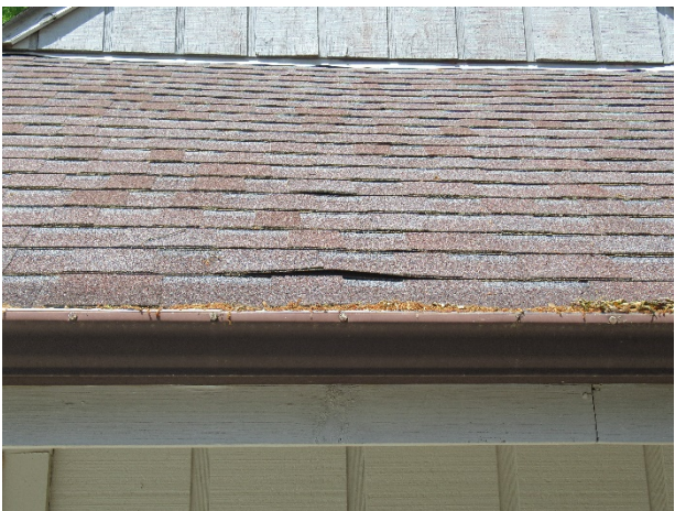
Pool house shingle lift
