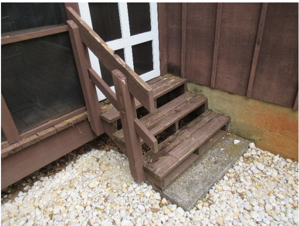
Stairs with railing at southeast deck
