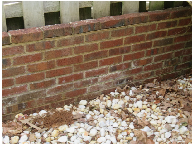
Efflorescence
