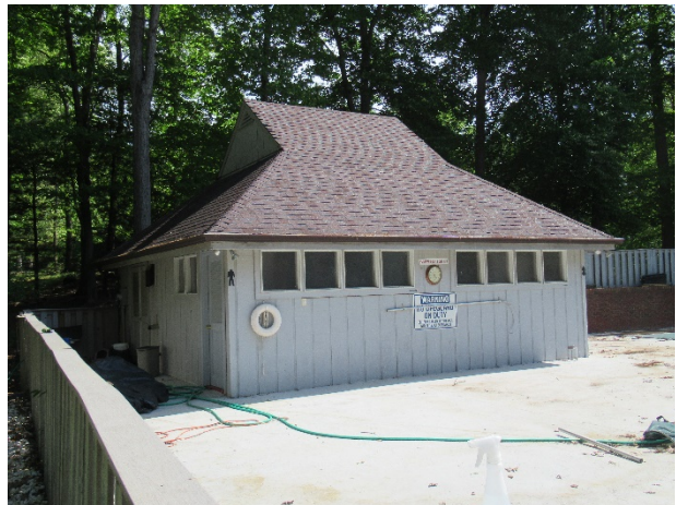
Pool house roof overview
