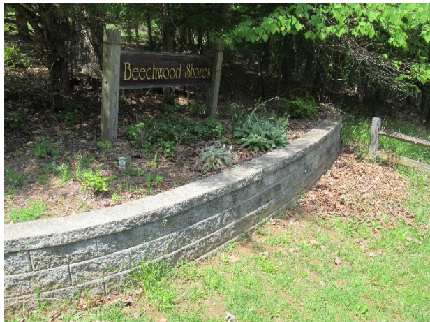
Retaining wall overview
