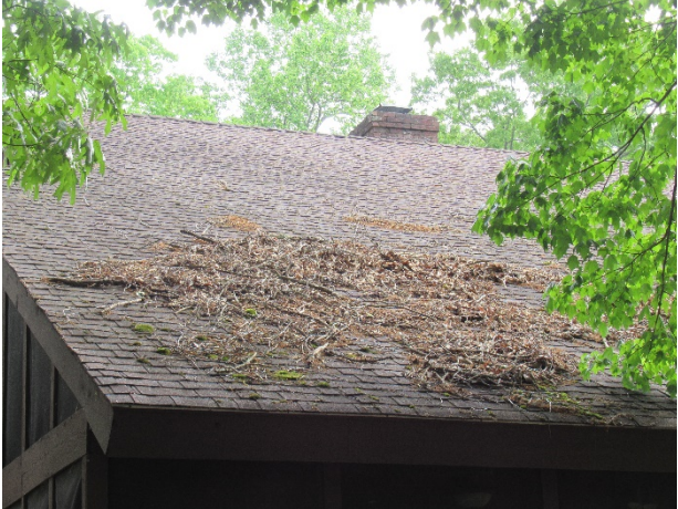
Clubhouse roof overview
