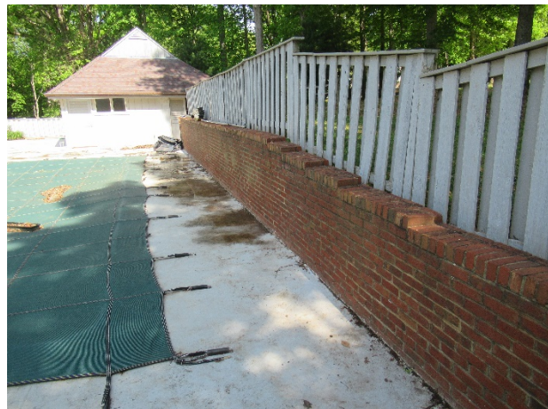
Masonry retaining wall overview
