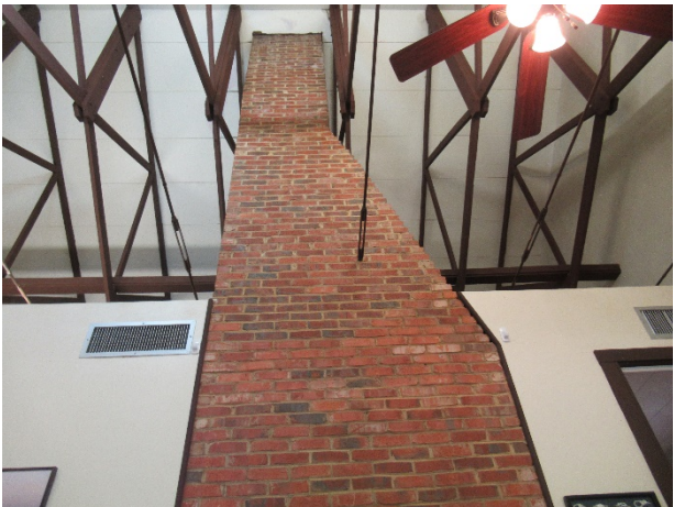
Masonry fireplace overview
