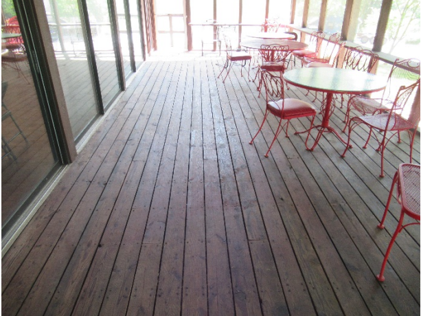
Wood deck overview at southeast elevation
