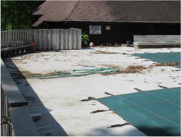
Concrete deck overview
