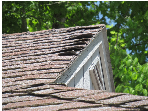
Pool house shingle lift
